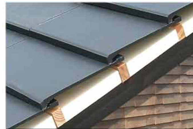
屋根外断熱工法 Air-roof insulation system
